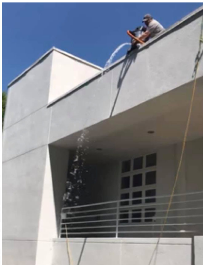
Anibal flushes a drain on our roof.
